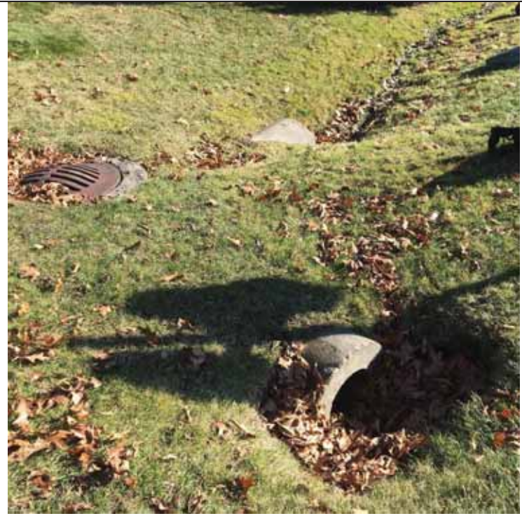
Beehive CB on Steeplechase. Connects Rd drain ditches. Flow in E. ditch line. Sampled
