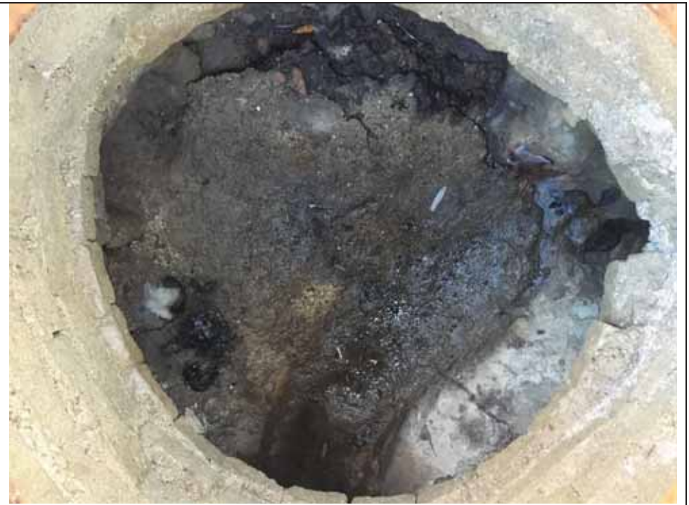
local storm MH for connected Rd drains on E. side of Charring Cross. Dry w animal feces
