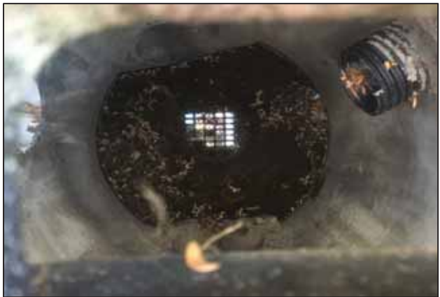
Inside of catch basin.
