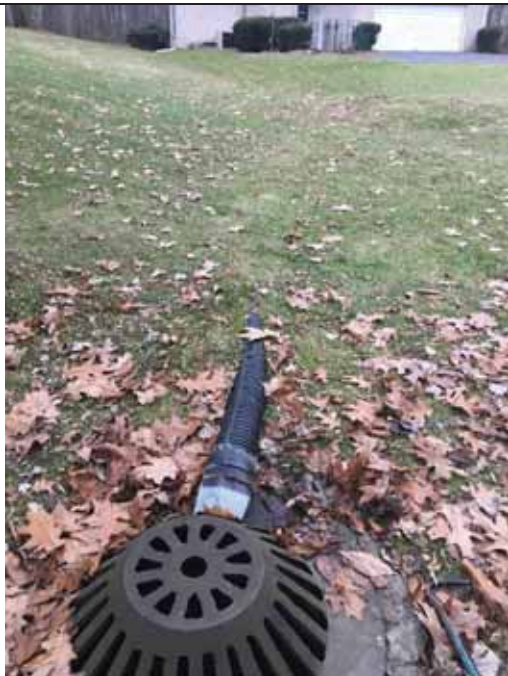
Plastic PVC drain from 482 Whippers LN connected to Back Yard CB Beehive. No flow.
