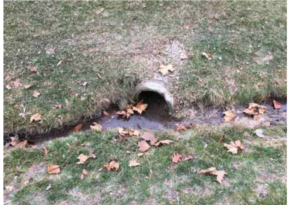
Drainage Ditch N. of MH 408. Flow is clear. Inlet pipe in ditch connected to MH 410.
