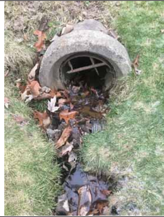
Inlet to CB 13369 w flow from drainage ditch to the W. Flow is clean
