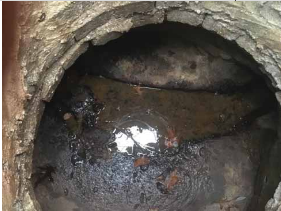
MH 7318 Connected to MH 407. Animal Feces on MH floor and channel. Sampled
