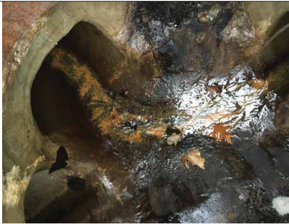
MH 407 flow from N. Rd drain inlet E. is dry w/ animal feces in MH. Sampled
