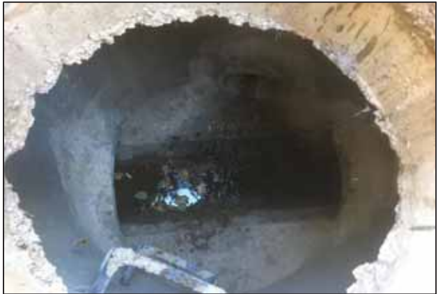
Outfall is east invert (top of picture)
