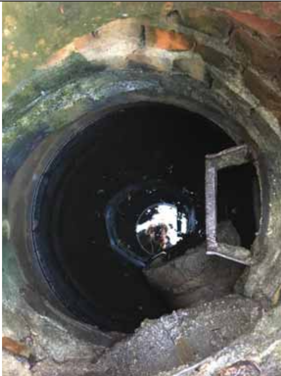
MH on Hunt Master. Connects Rd drain ditches to drain. Water in CB sump. Sampled
