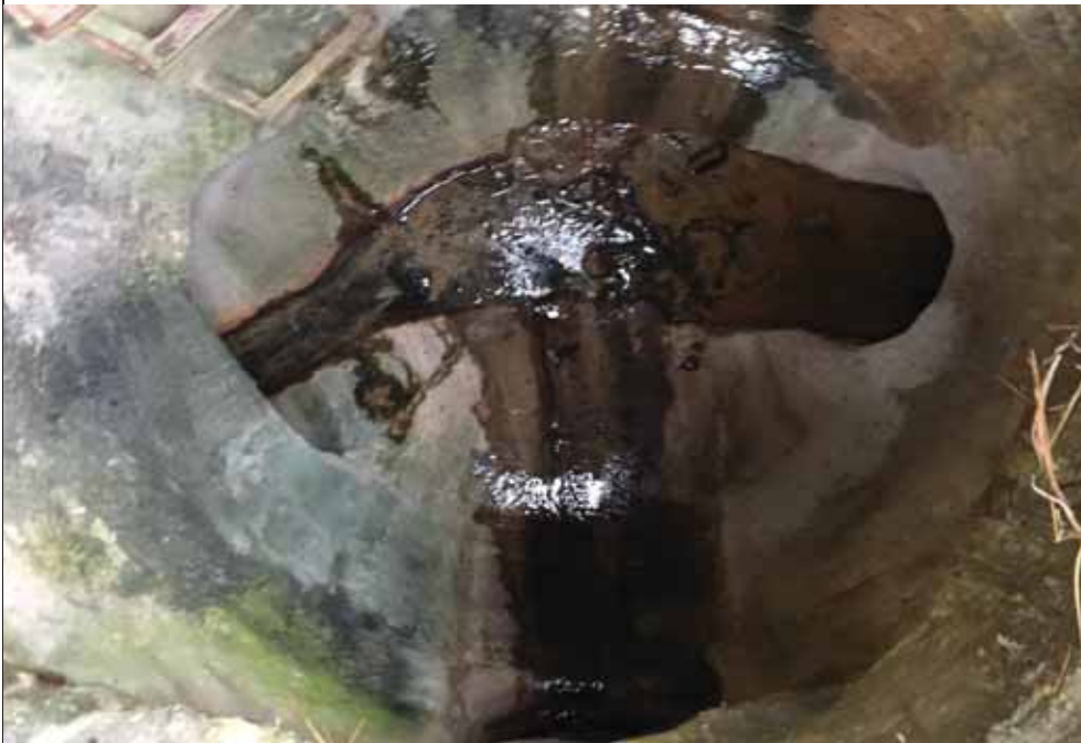
MH 408 . Flow from N. is pooled at elbow going E. Brown with suds, staining on MH wall
