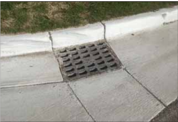
Catch Basin within Exeter Road
