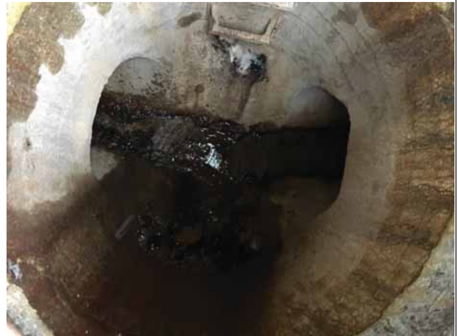
MH 410 – Connecting MH CB B 13378 to drain going E. Animal feces in MH. Sampled
