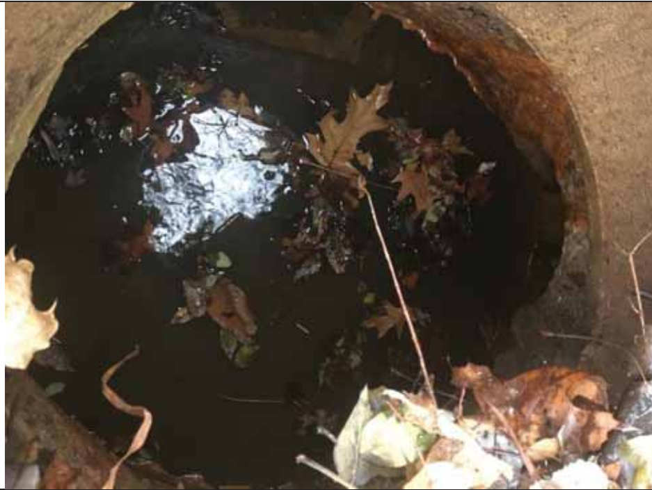
CB 13369 connected to MH 7317. Inlet flow from ditch line W. Looks clean. Sampled
