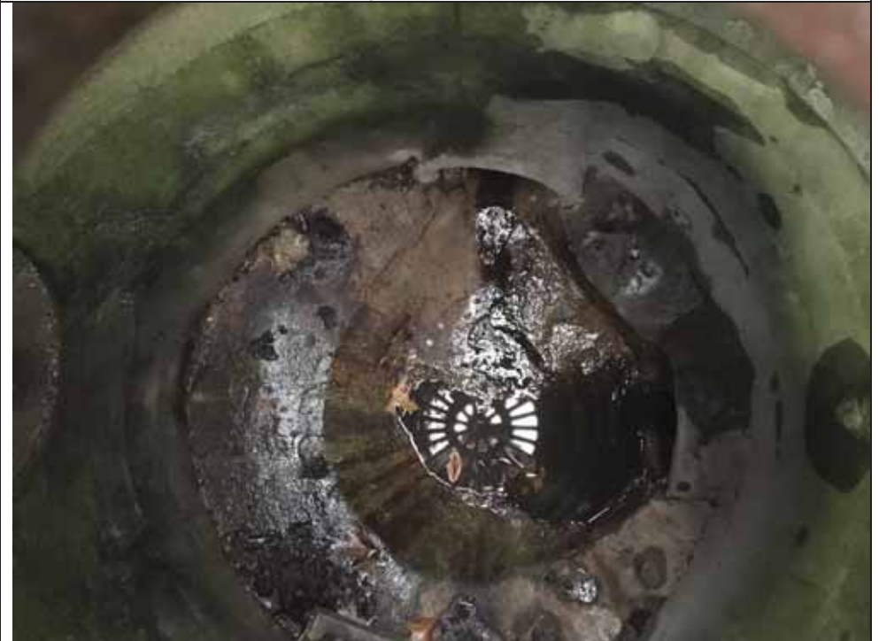
CB connects inlets for Whippers LN. & Hunt Master to MH 7316. Ponding at E outlet
