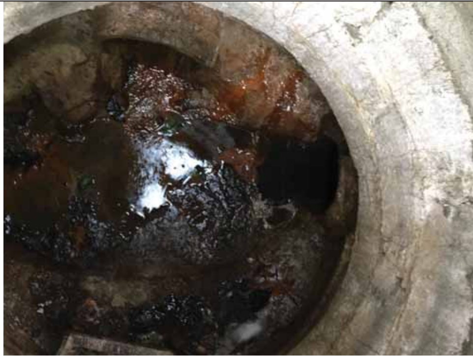
MH 7316. Terminus MH. Connects local drains W.& S. Sewage and animal Feces in MH
