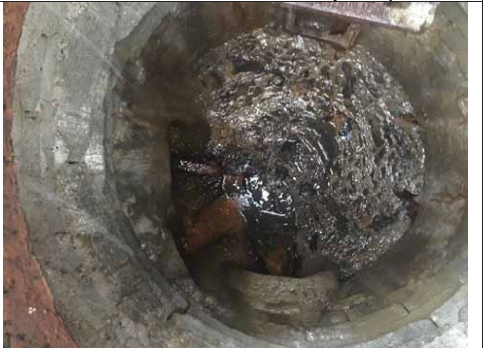
MH 7317. Elbow from W. to S. Possible sewage in MH. Sampled. Connected CB to the S.
