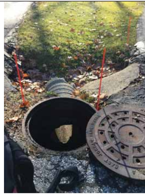
MH on Whippers Lane. Connects Rd drain ditches to drain. Water in sump. Sampled
